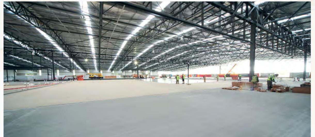
Commonly known as 'Project Century', Lion Nathan brewery situated in South Auckland is built to last for 100 years. Constructed with a focus on quality and longevity, floors for the facility were installed with Ucrete DP heavy duty PU-hybrid system to meet the performance expectations.
