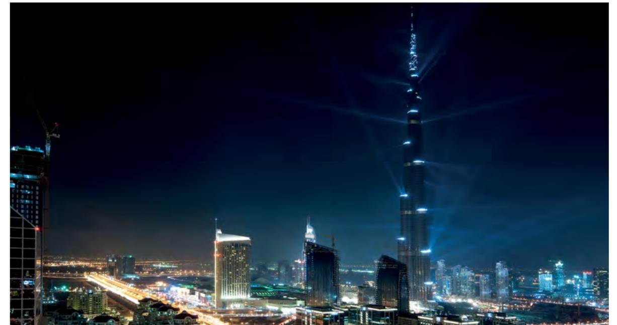
Burj Khalifa, the tallest tower till date standing at 828 meters high. Master Builders Solutions developed a concrete mix that can be pumped to a height of >600 meters without interruption, to shape the structural form of the tower. Withstanding high ambient temperatures without segregating, MasterGlenium Sky admixtures
